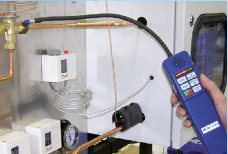
Leak testing at expansion valve
