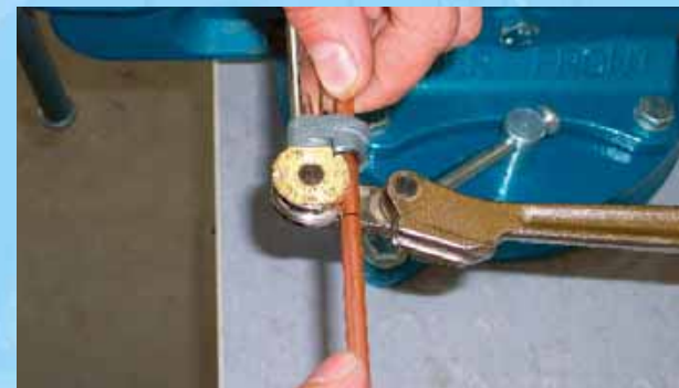
Inserting the pipe into the bending device
