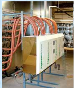
An example from practice: industrial air conditioning system with comprehen- sive filters for clean room production
