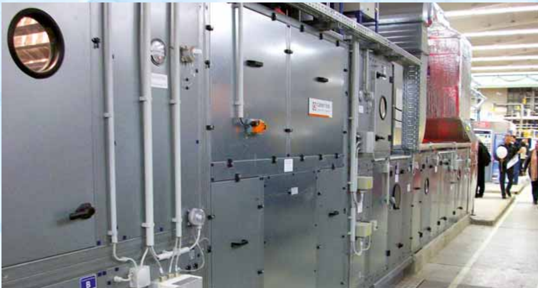
An example from practice: industrial air conditioning system with comprehen- sive filters for clean room production
