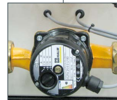
Non-controlled circulation pump with selectable speed (efficiency class C)
